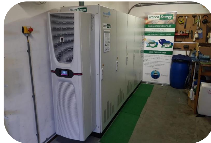
120 kWh - Time Shift energy storage
